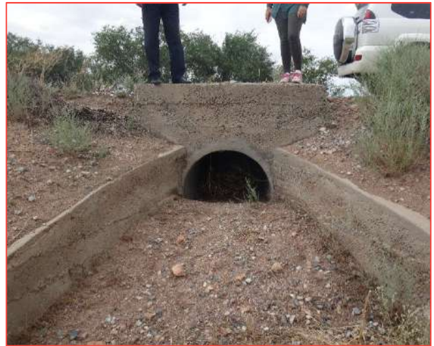
Figure 5 - Typical Drainage Pipe
